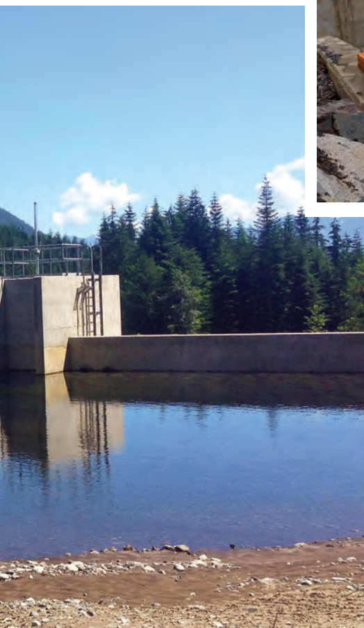
Right: Marty Creek main intake, showing Coanda screen and maximum diversion control weirs.
