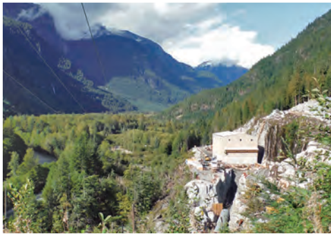
Top: Diversion weir with 20m-long inflatable rubber dam that deflates in a flood event. Inset: Built on an elevated rock platform, the power station houses two vertical axis pelton turbines.
