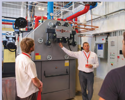
Demonstration of the commercial biomass wood-fired boiler, led by Andreas Wintzer of Viessmann.
