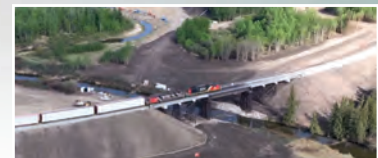
May 15, 2016 - Rail service is restored
