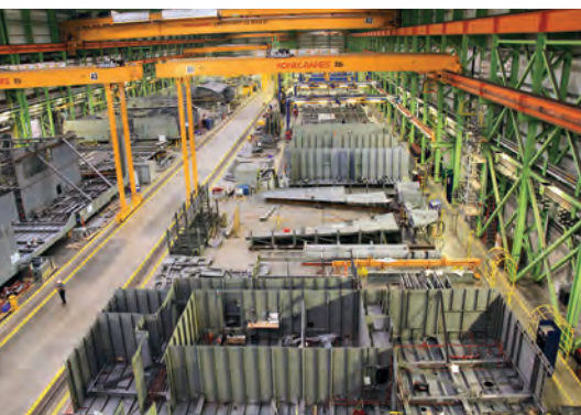
The shipyard modernization project was a complete redevelopment of Irving Shipbuilding Inc.'s facility in Halifax. Inset: The Assembly Hall is a 265m-long structural steel production hall.
