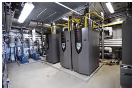
Top: Mini-plant installed on parkade roof behind sound wall structure. Inset: District energy mini-plant interior layout.
