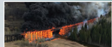
April 26, 2016 - Bridge destroyed by fire
