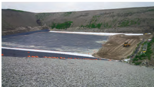
Top: Waste screening operations. Inset: Construction of the final phase of geosynthetic liner.
