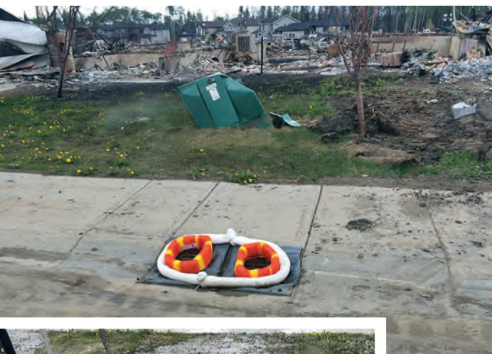
Clockwise from top left: Silt socks and erosion barriers were installed on catch basins in the devastated neighborhoods; Sewage service connection “Cut and Cap” initiative for monitoring and cleaning the siphon headworks vaults; Each catch basin was then photographed and tagged in the GIS system.
