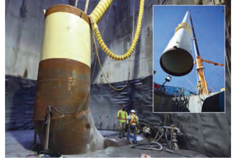
Pipe elbow at bottom of shaft. The pipe is supported only at the bottom of the shaft and at the valve chamber end wall—a 60-metre span.
