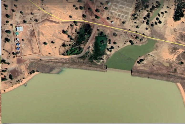
Drinking water supply
